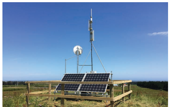
WISPs use thousands of radio sites like this to bounce Internet signals from hilltop to hilltop at city speeds throughout rural New Zealand.
